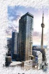
87 Peter Peter & King Under Construction
